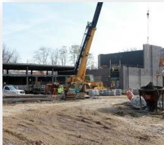
E.V. Moore Building Additions Under Construction April 2015
