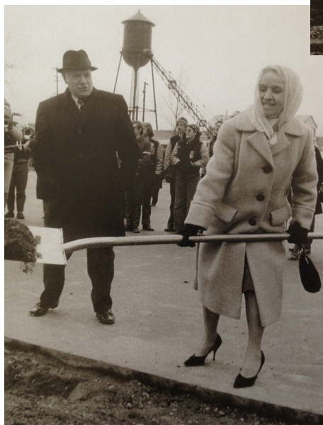
WILLIAM D. REVELLI LOOKS ON AS MARY REVELLI TAKES HER TURN AT THE GROUND-BREAKING CEREMONIES
